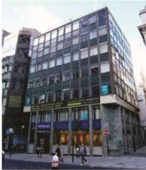
Front elevation looking north from Cannon Street
