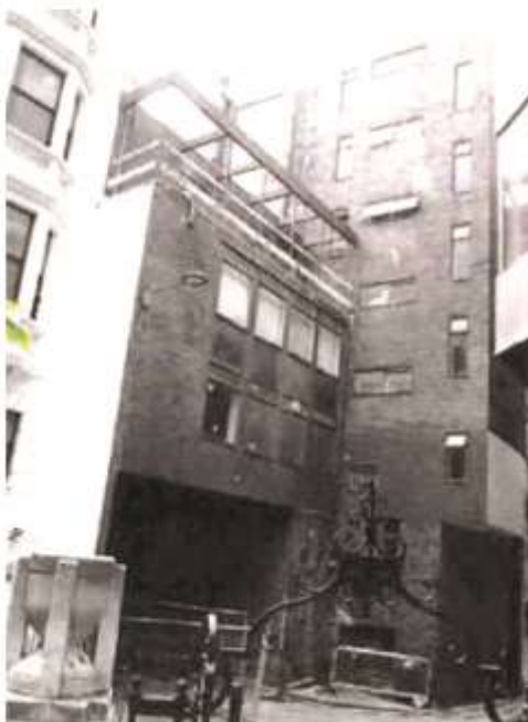
Rear elevation in Salters Hall Court looking south
